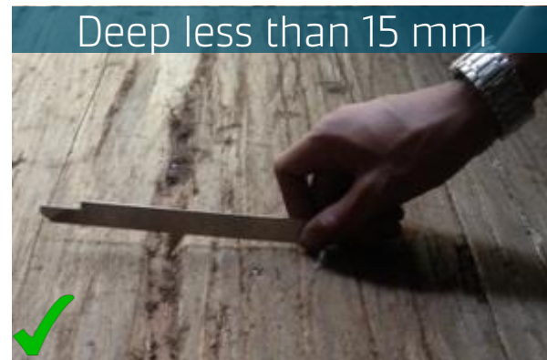
Illustration 2: Gouge on floor
